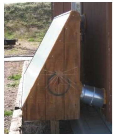
Side view of solar heating system, showing ducts for air intake and return
