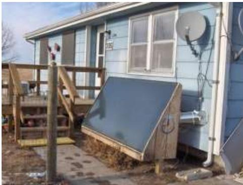
LSE's solar heating systems are manufactured in its facility at Pine Ridge. The main component of each unit is a four-by-eight-foot solar collector panel, made of a black metal film covered by a sheet of special solar glass and surrounded by a metal frame.
